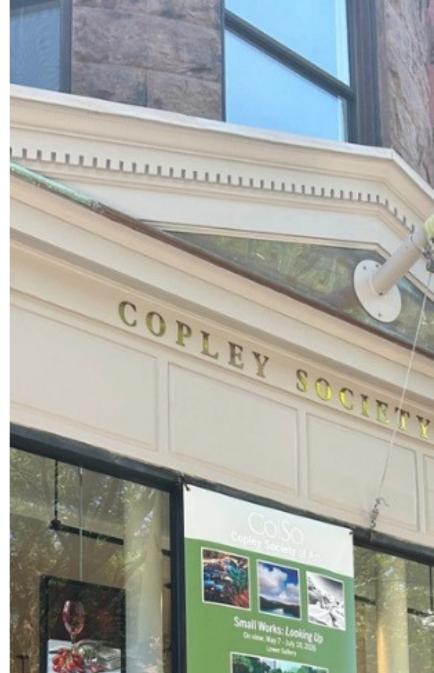
Our renovated facade at 158 Newbury Street
